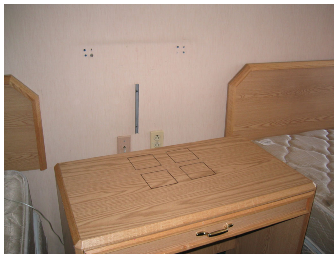
Figure 3. Horizontal wipe sample location D showing the 4 – 100 cm 2 sampling locations.
