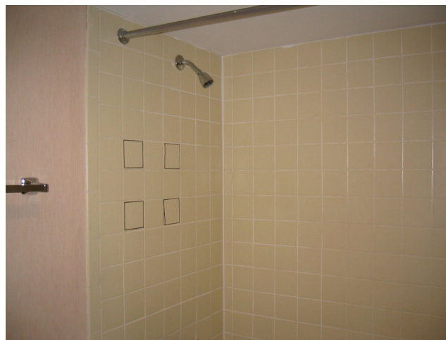
Figure 4. Vertical wipe sample location F located in Bathroom shower.
